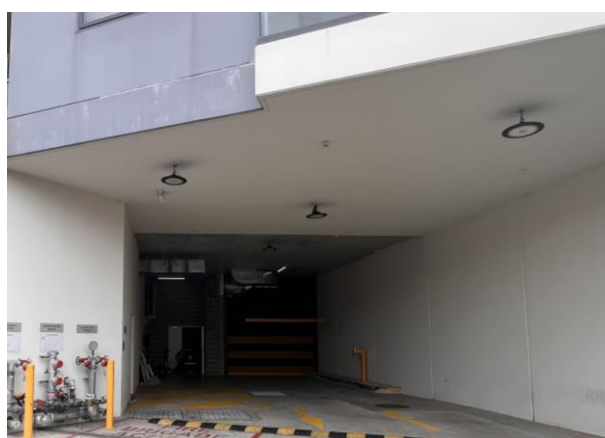
Potential Inundation at Carpark Entrance on Rodd Road, near Great North Road
