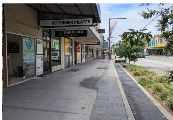
Stormwater drainage on Great North Road near Ramsay Road.
