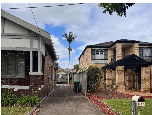
Area of overland flow between house at downstream end of Lyons Road West
